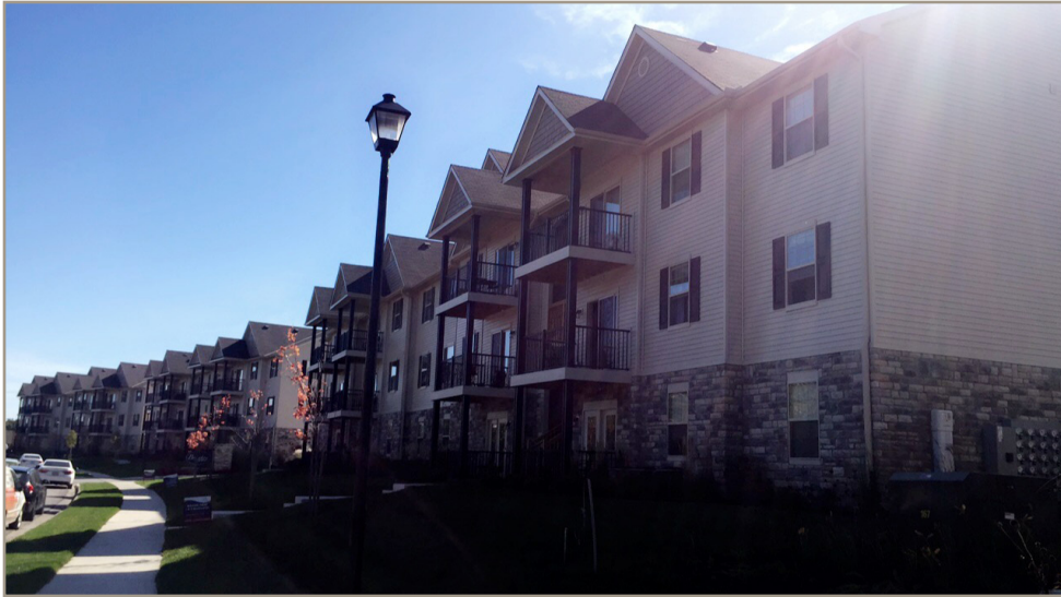
Apartment developments on the Northwest side.
